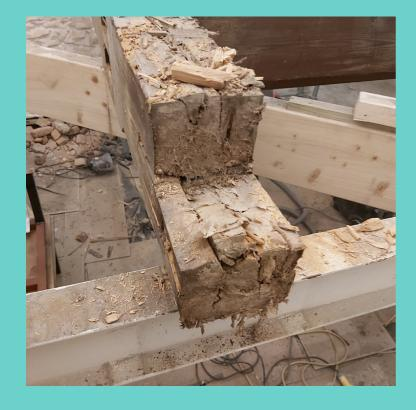
Work has been ongoing ever since with all the rotten wooden beams being removed and the internal walls being treated for the effects of the dry rot. The work will continue over the next few weeks to replace all the wooden beams with steel girders and reinstate the organ loft ceiling and the ringing room floor.
